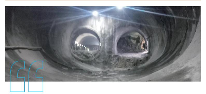
The Sahar Road Crossover Cavern (SRCC) is a tunnel with 6 symmetrical cross sections on Mumbai's Metro Line 3. The SRCC's original design called for a conventionally reinforced, cast-in-situ secondary lining. However, due to its complexity, Mumbai Metro Rail Corporation explored the use of sprayed waterproofing membranes (PSCL) and a drained regulating layer.
