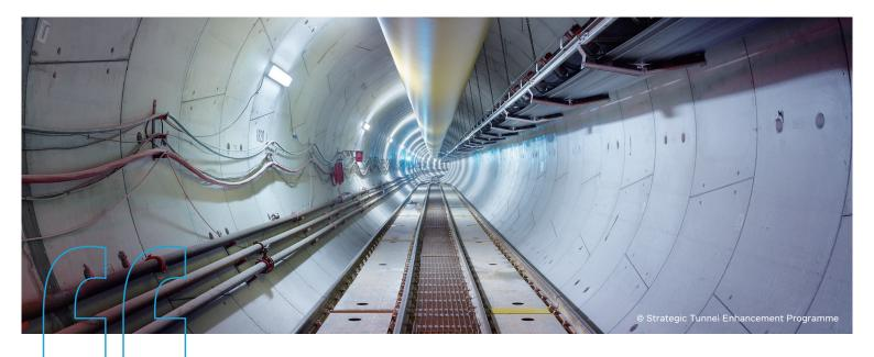
Abu Dhabi's Strategic Tunnel **Enhancement Programme** (STEP) is a deep gravity wastewater sewer system. The size and scale of this megaproject was groundbreaking for the region, deploying seven TBMs at depths down to 80m. The robust tunnel system has provided a sustainable solution that reduces the agency's operating budget and carbon footprint, as well as improving the local environment.
