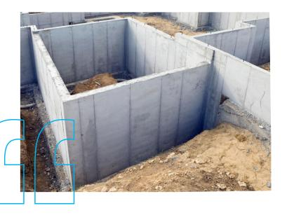
A cellar wall is a specialized precast concrete element designed for subterranean applications, primarily used in building foundations and basements. Cellar walls are essential for creating stable and secure underground environments, offering enhanced strength and durability when reinforced with our Dramix® steel fiber technology.
